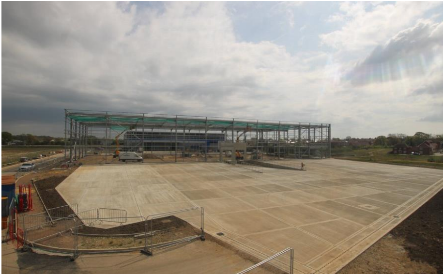
Time lapse camera view of the external yard and building footprint
